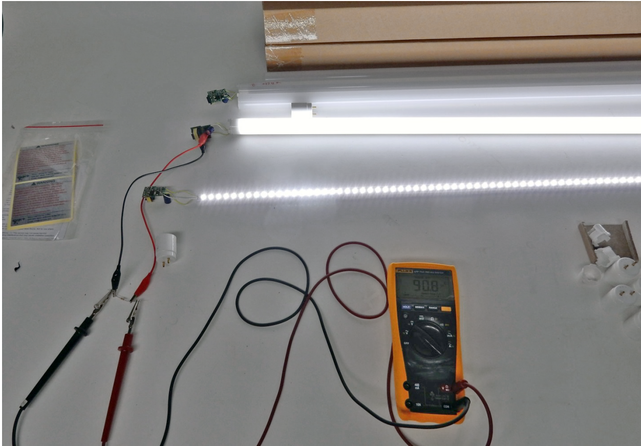
Figure 4: Lamps restored to proper operation
